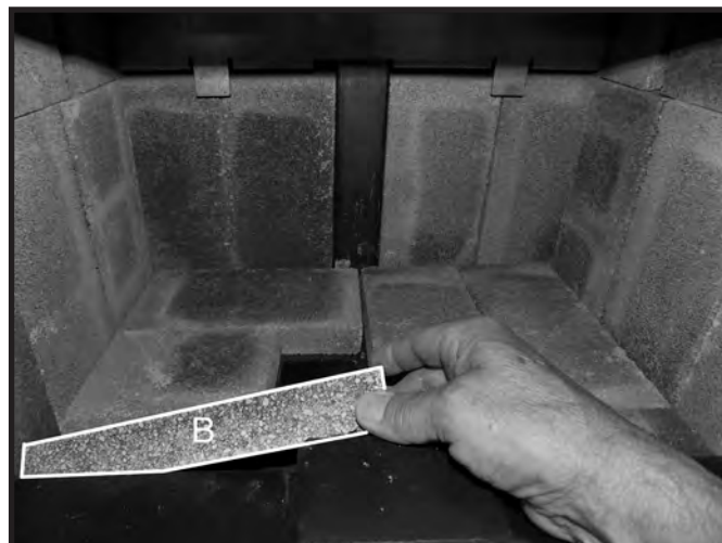
Figure 30: Final narrow brick in place.
